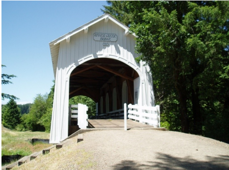
Bricks are being placed in the walk at the south end of the bridge. The next batch is on sale.
