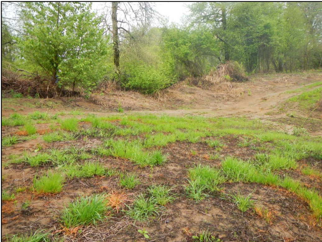
Figure 4-2. At SIA #8, the existing access road is set at the same elevation as the invert of the swale. The bank elevation could be lowered slightly to allow floodwater to access the swale and the pond located to the north.
