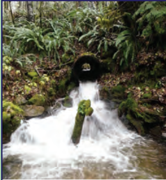
Culvert outlet, pre-project (2019)
