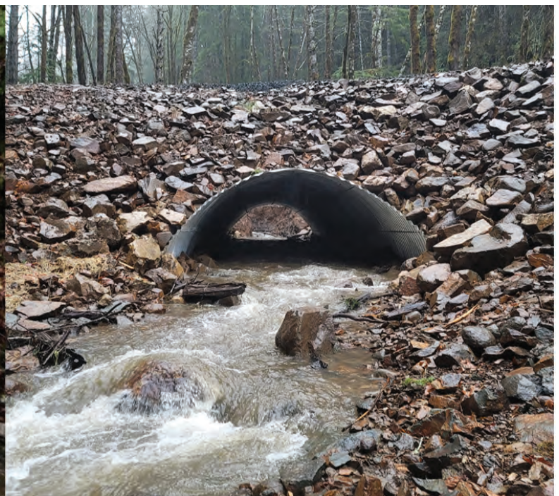
Right: Upper culvert outlet, post-project (2022)
