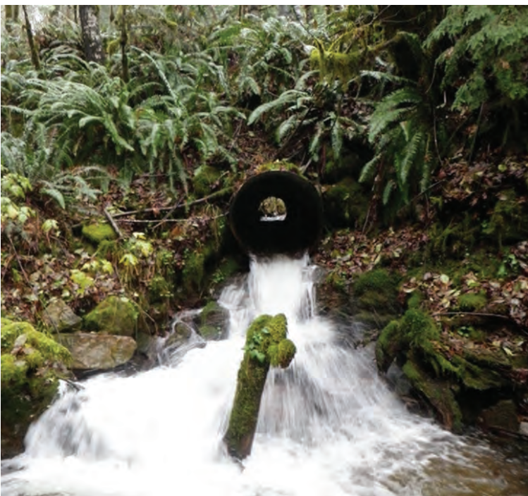
Left: Upper culvert outlet, pre-project (2019)
