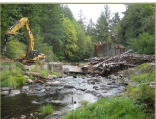
Contractors work on the Luckiamute River Bridge Piers Modification
