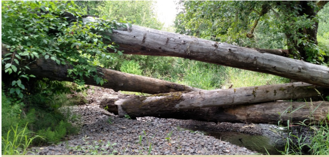
Because it provides many benefits to fish, "large wood" placement is an important part of many of our stream restoration projects.
