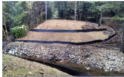
Sep. 2013: Post-project view of berm, showing new side channel. J.P. Zagarola
